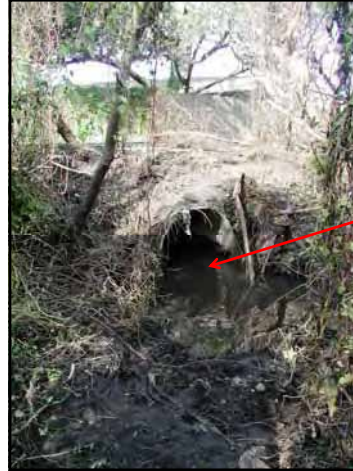
1/19/2006 Mud and debris removed from marsh at culvert outfall.
