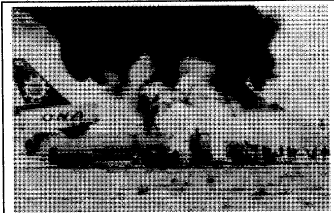
This DC-10 was destroyed by fire when several herring gulls were ingested into an engine during takeoff from JFK International Airport, November 1975 (see story on page 17; photo courtesy Port Authority New York and New Jersey).
