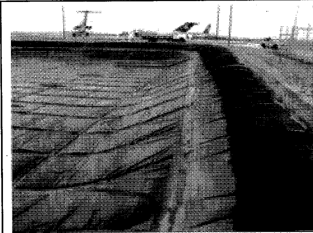
Birds are permanently excluded from this storm water detention facility through the use of a floating permeable barrier (Photo courtesy Industrial & Environmental Concepts, Inc.).
