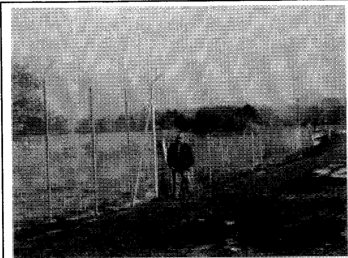
A well-maintained fence, at least 10-feet high with no gaps at the bottom, is the primary defense to keep deer and other large animals off the airport's AOA. Deer can easily jump fences that are only 6 feet high (right) (photo by R. A. Dolbeer, USDA).
